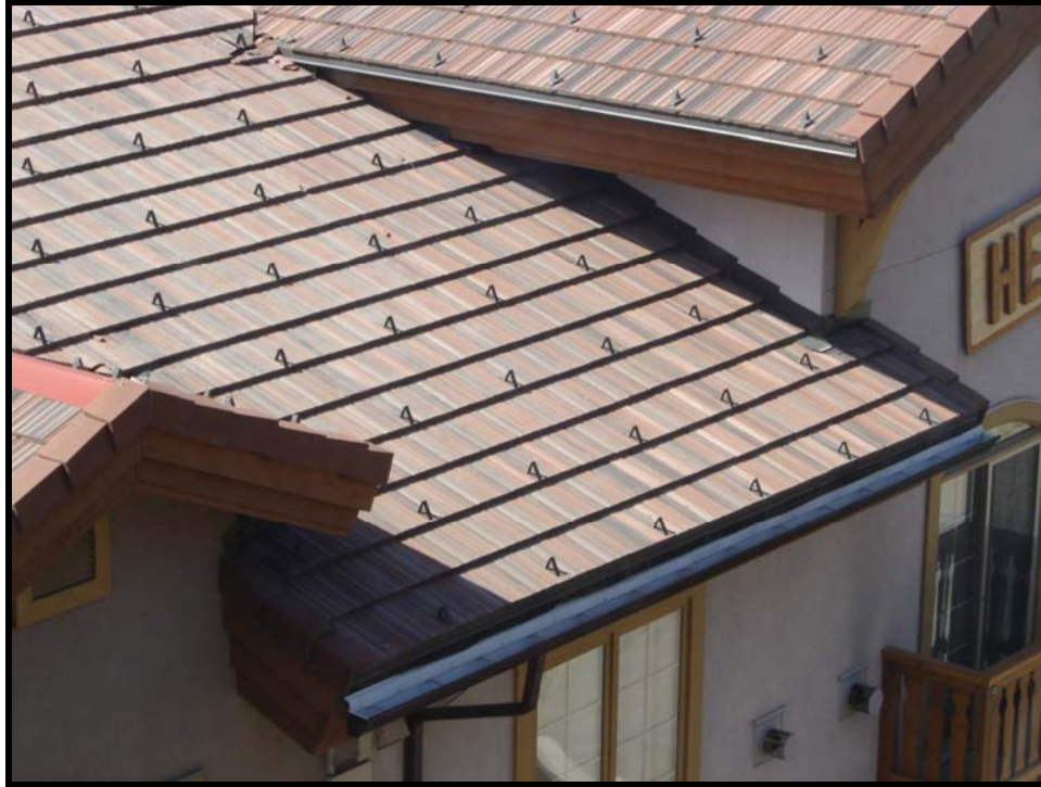
Roof Surface and Snow Clips – Village at Sun Peaks
