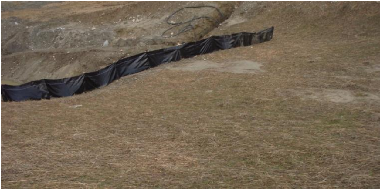
Sediment fencing and soil erosion protection
